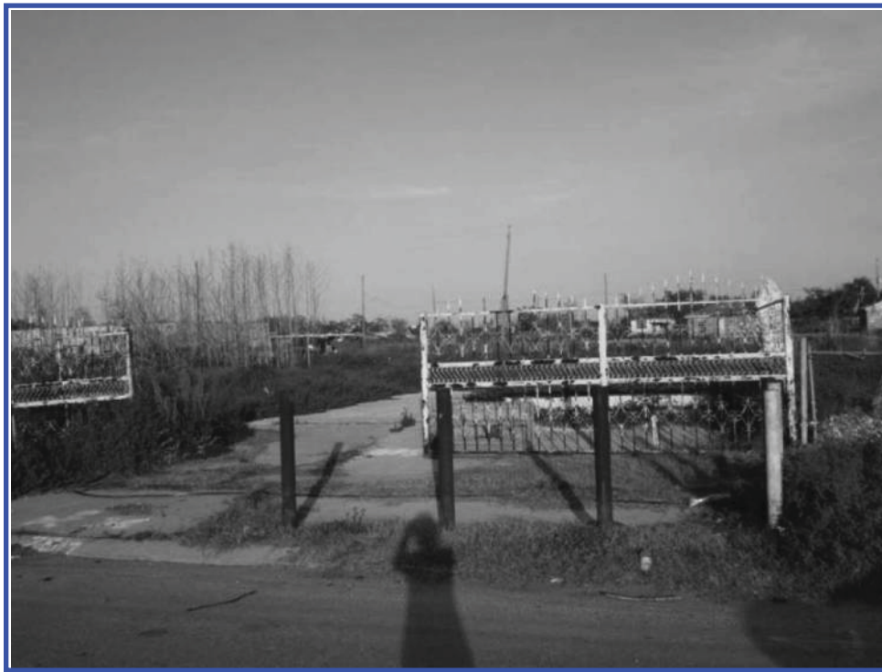
Figure 3. Lower Ninth Ward demolition site, 2008. Photograph by S. Dawdy. A color version of this figure is available in the online edition.
